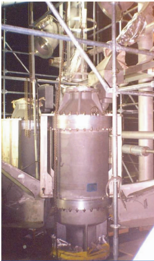
Figure 1. A submerged motor cargo pump being installed inside an LNG carrier.
